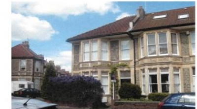
A different front bay and roof treatment
