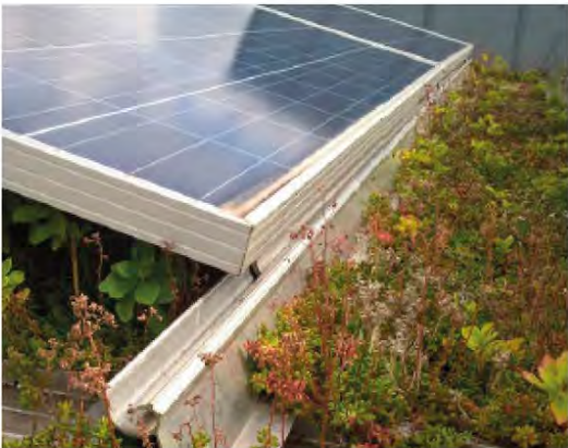
Bio-solar living roof
